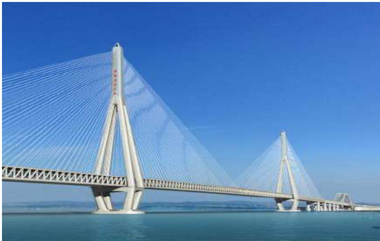
Span: 1208 m, height of main tower: 350 m
